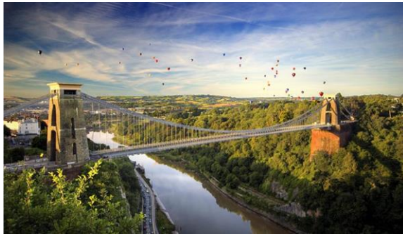
13 Clifton Suspension Bridge (Bristol)
