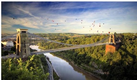
13 Clifton Suspension Bridge (Bristol)
