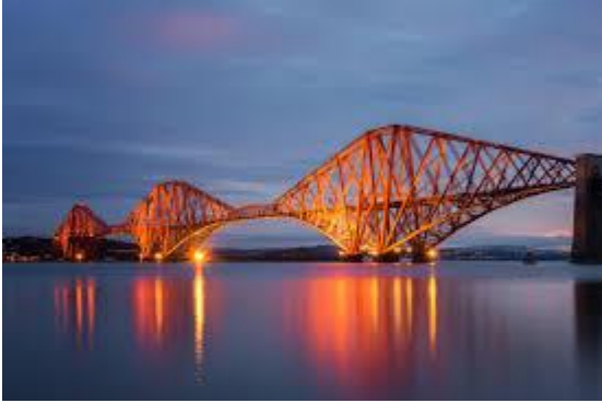
1 The Forth Bridge
